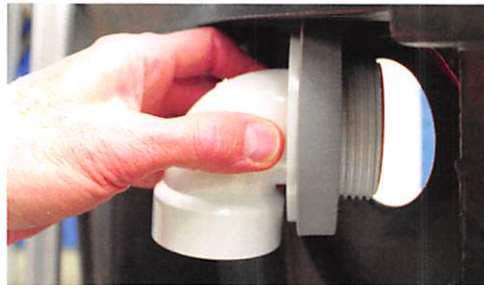
Overflow ell extends through hole
